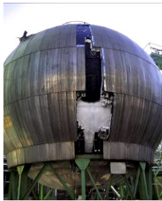
Superficial damages suffered by a NH 3 tank
