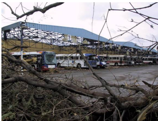
Bus depot destroyed
