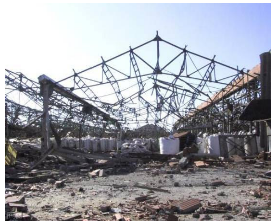
Warehouse destroyed by the blast
