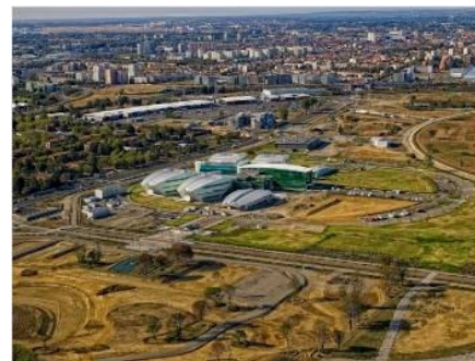
The cancerology center under construction (source : Oncopôle Toulouse )
